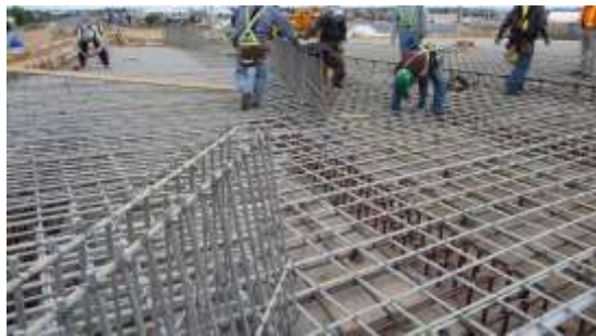
Fig. 2: FRP decks/app slabs/ barriers, Skagit River – BC MOT (2009).
