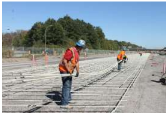
Fig. 5: GFRP bar placement in center lane in Highway 40 (Montréal)-2013.
