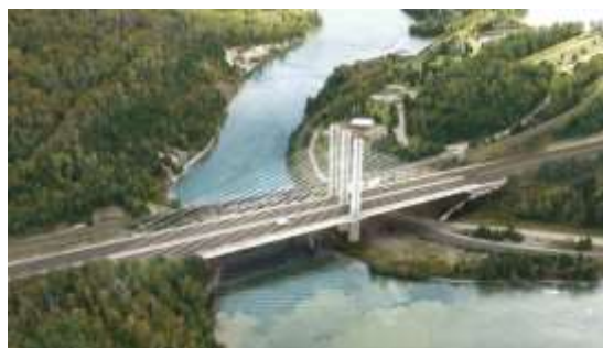
Fig. 3: Cable stayed bridge, Nipigon River Bridge, ON (2015).
