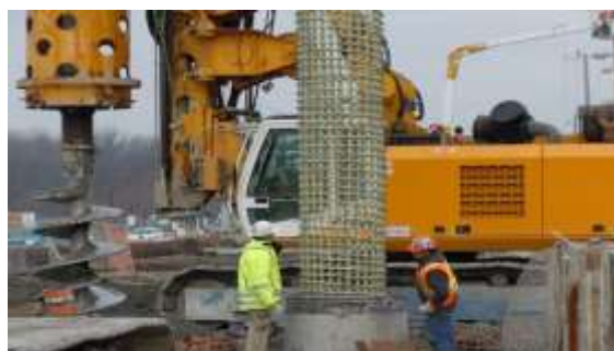
Fig. 4: Handling and lifting the GFRP Soft-Eyes.
